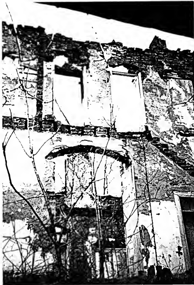
Figure 26: Interior masonry wall of addition
